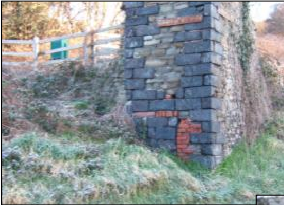
Plate 4 Close-up of chimney base
