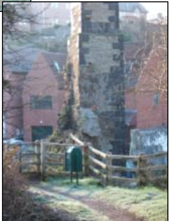
Plate 5 Close-up of chimney base
