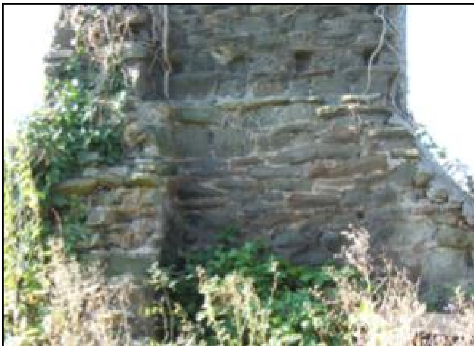
Plate 6 Close-up of chimney base
